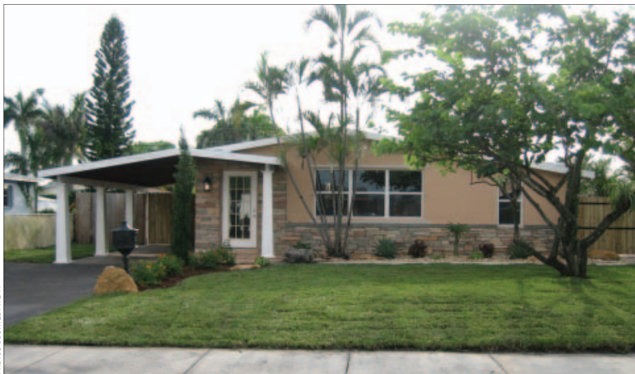
This former "Ugliest House on the Block" in Oakland Park, Fla., got a hurricane-friendly makeover, including a LEED certified, cultured stone veneer wainscoting from Owens Corning and Energy Star windows. Landscaping packed with water-retention liquid crystals reduces watering.
